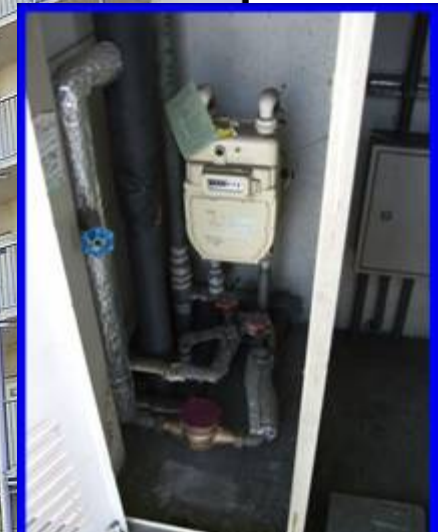
Internal of pipe-shaft
