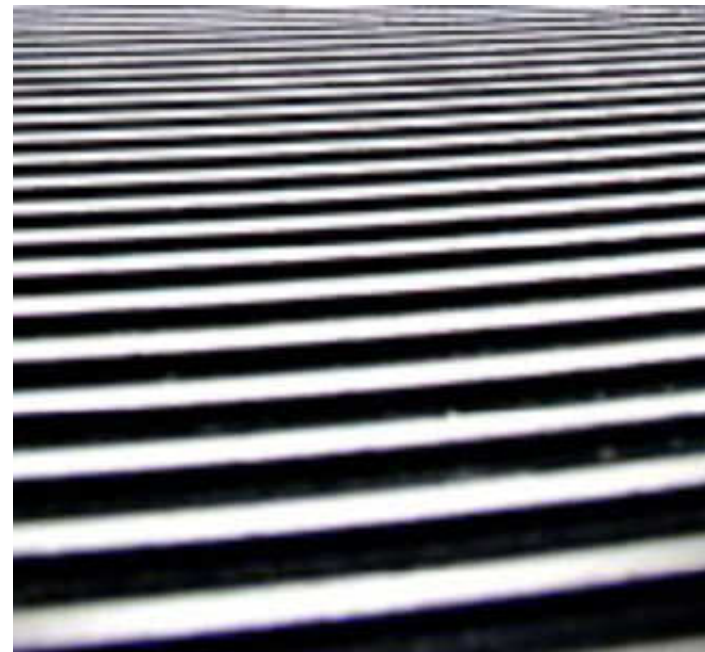
Escalator stair tread [Wilkins, 2009]
